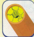
Sludged up pipework
